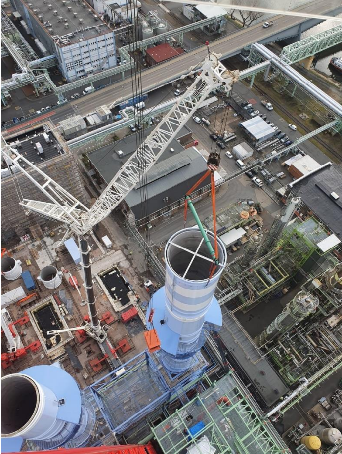
Bypass stack erection
