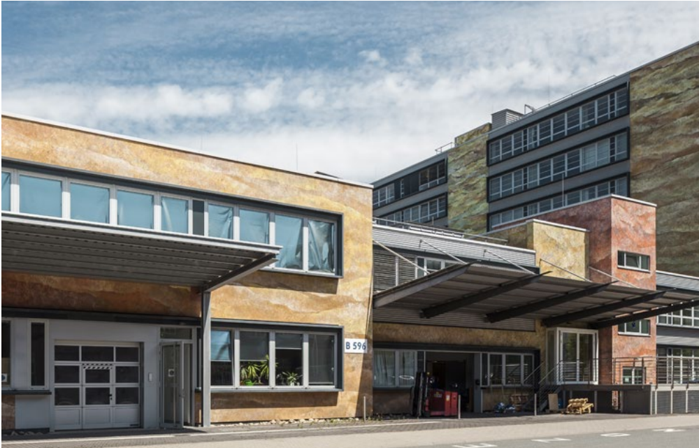
South view with delivery entrance
