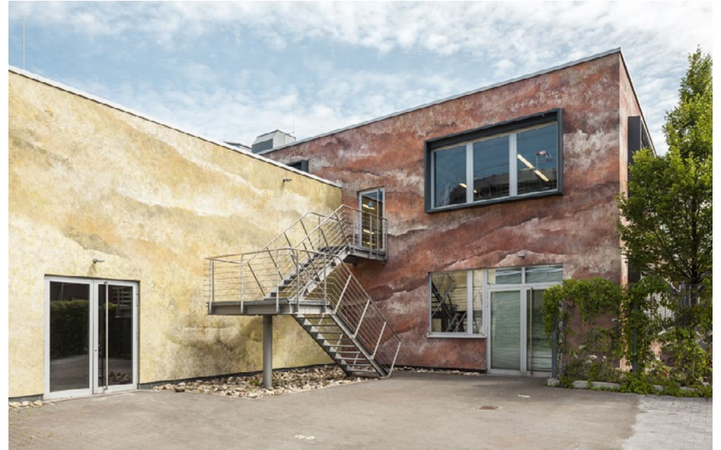
Southwest emergency exit
