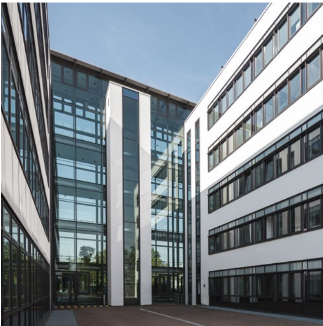
View between Building Modules G877 and G875
