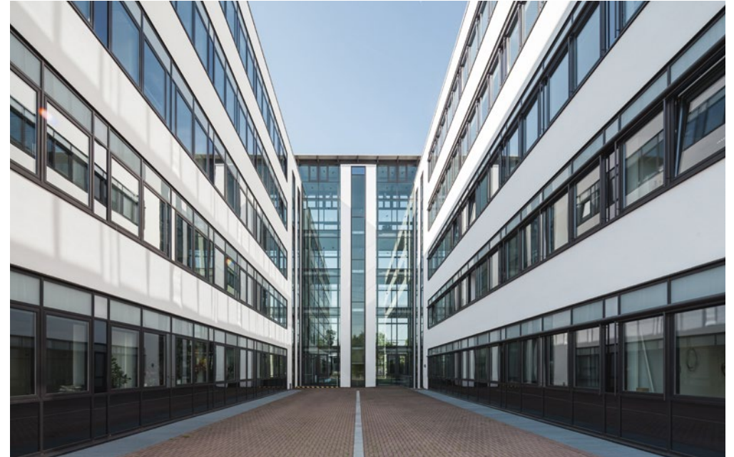
View between Building Modules G877 and G875
