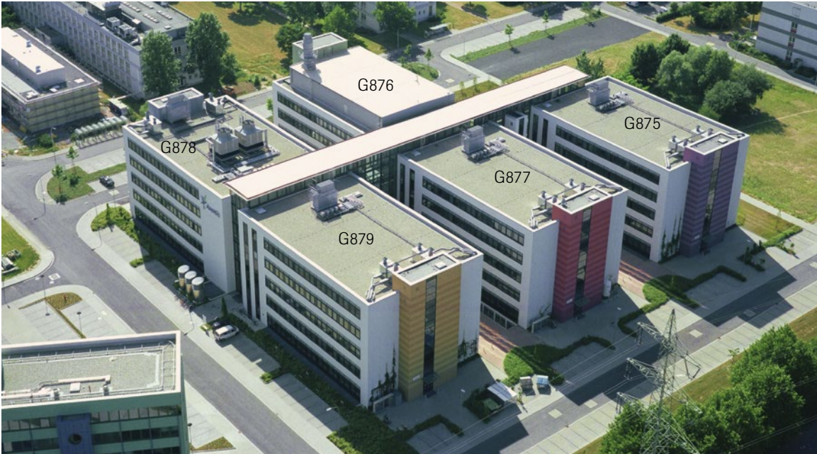
Bird's eye view of the multi-purpose laboratory building (from the southeast)
