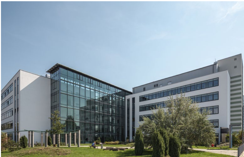
The brightly lit central block in the northeast corner of the building with a small park. It connects the five building modules.
